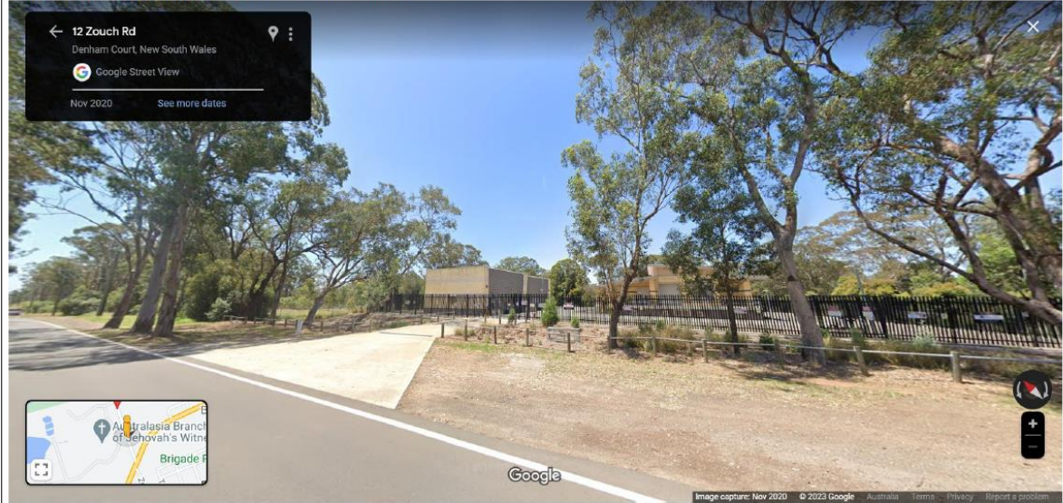
Google Maps Street View. Edmondson Park Zone Substation.
